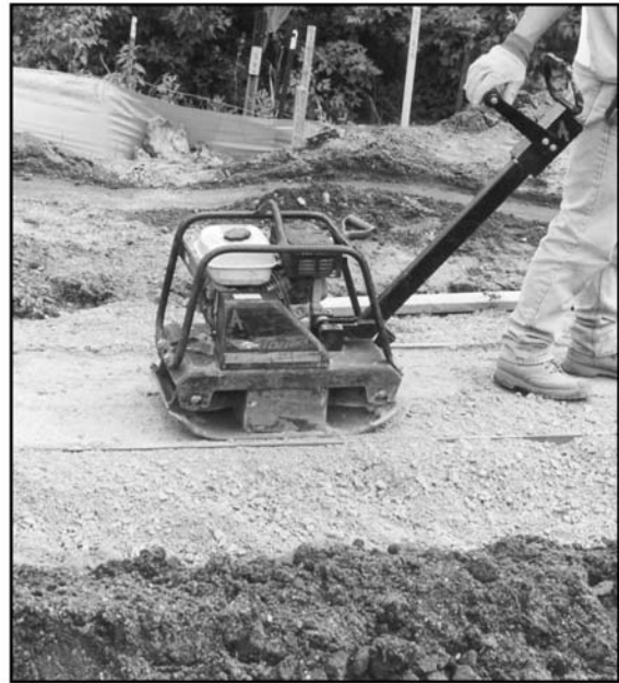
Compacted granular leveling pads provide a stiff but flexible base.
